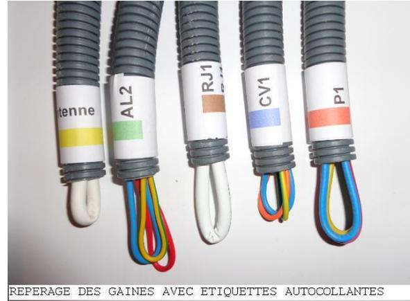
REPERAGE DES GAINES AVEC ETIQUETTES AUTOCOLLANTES
